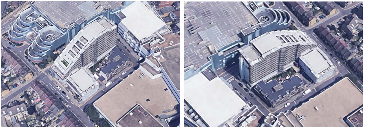
Images 2 and 3: birds eye views of the existing building
